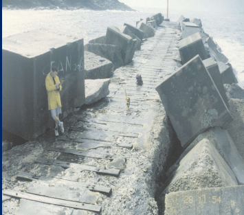
Coffs Harbour Head Storm Damage May 1997 12 x 40 tonne blocks
