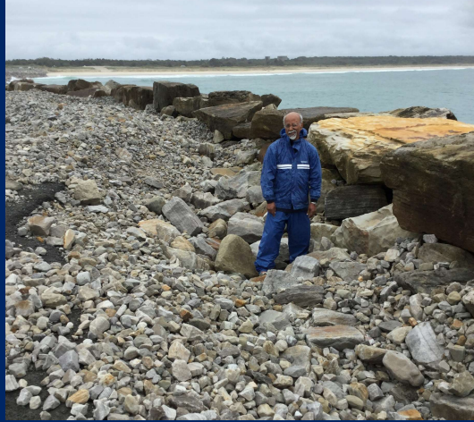
Severe Crest Damage at the North Clarence Breakwater – June 2016
